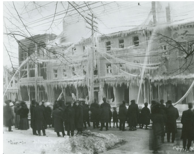
Fig. 4 1912 Barrington Street, looking east
