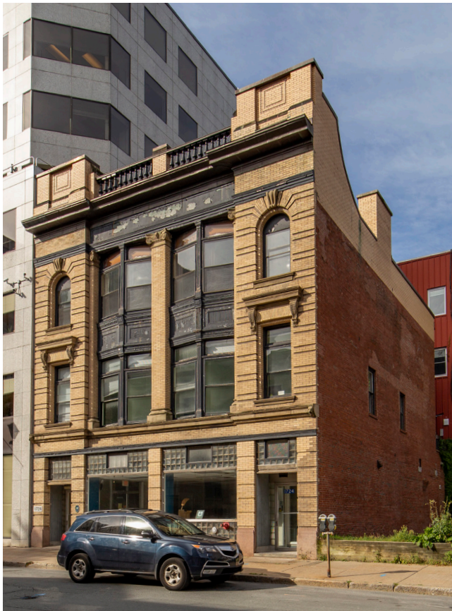
Fig. 16 Layers of site history are evident in the masonry changes on the exposed west wall of the Dennis Building
