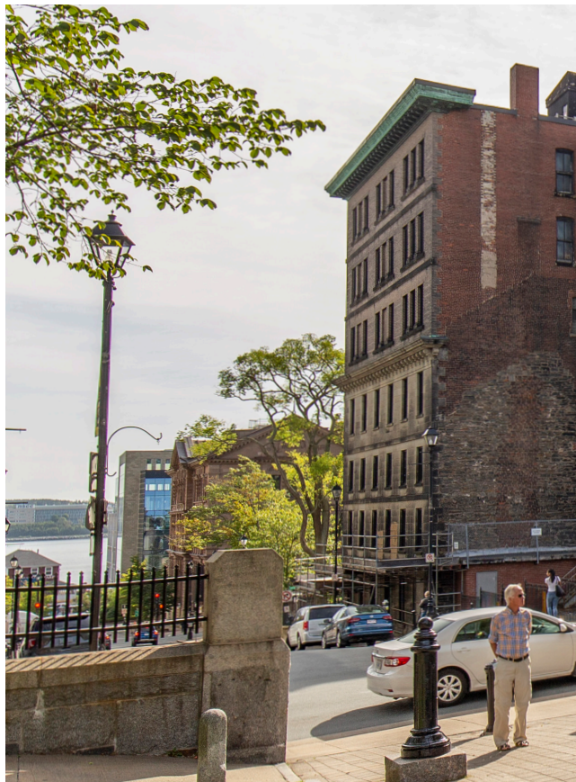
Fig. 14 Layers of site history are evident in the masonry changes on the exposed west wall of the Dennis Building
