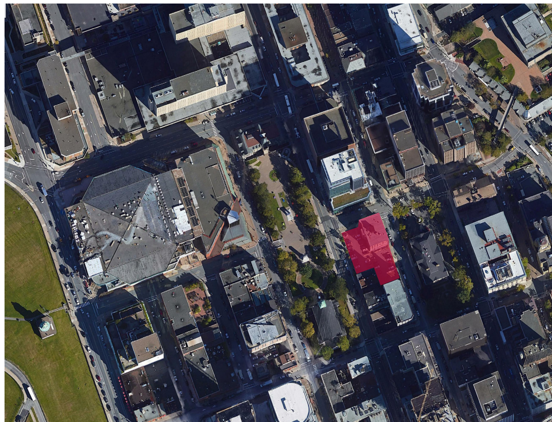
Fig. 1 Aerial map showing the Development Site location in red Source: Google maps, annotated by Fathom Studio
